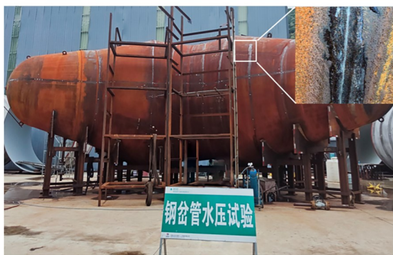
(a) 现场概况 (a) Site conditions
